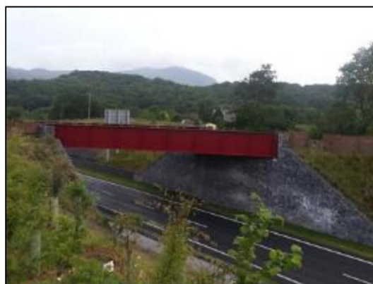
Figure E2. The environmental overbridge on the A487 from the southeast verge.
