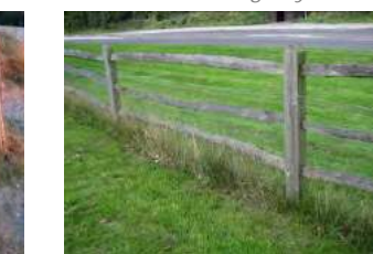
Hardwood post and rail fencing
