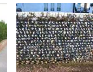
Flint wall with half round brick coping
