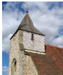
Shingles on church roof
